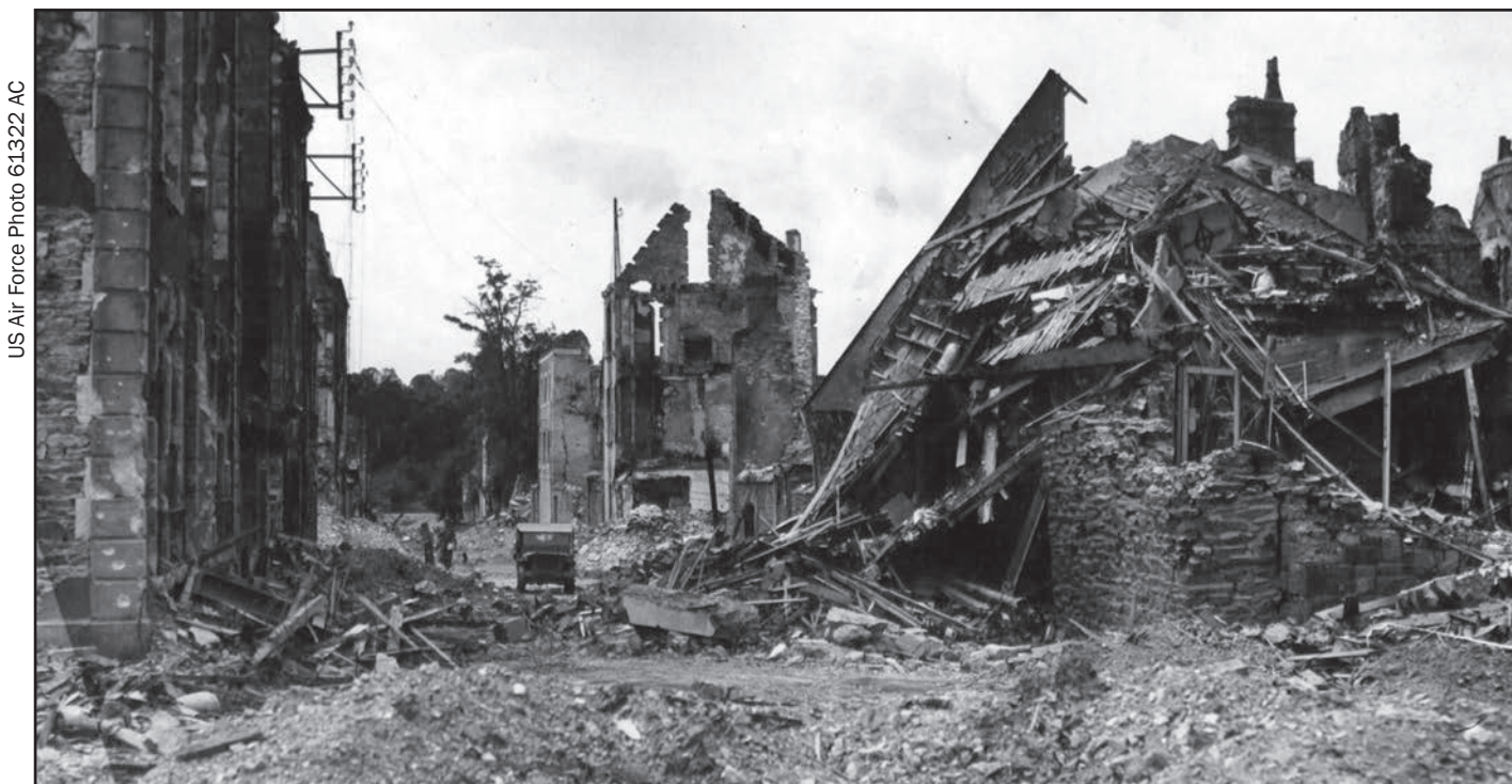
A US Army jeep is parked amongst the rubble of Saint-Lô following the capture of the city at the end of July 1944.
