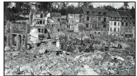
Above: Various ground views of the destruction in Lisieux.
